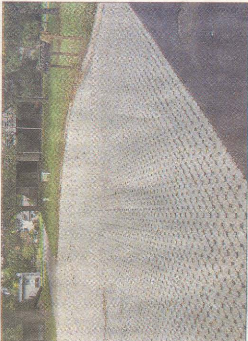
Porous pavers being used in a parking lot: In some situations, materials like these can reduce the amount of runoff that flows into rivers and streams.
